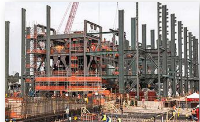
Construction of Vogtle Unit 3 Turbine Building,
